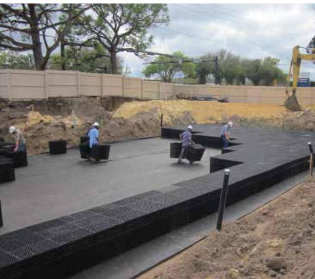
R-Tank is a modular system and can be assembled to a variety of heights from 2" to just under 7'. This rigid system can be placed beneath a variety of surfaces including: Parking Lots, Streets and Access Roads, Driveways, Landscaping, Athletic Fields/Playgrounds, Swales and Channels.
