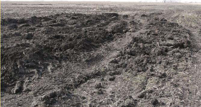
With a scraper you are loading your bucket every couple of hundred feet and then you have to pull out and drive away to unload it. This is a lot of turning, realigning and bouncing around in the cab. When you're done you have piles of dirt all over the field that need to be smoothed out as a second operation.
